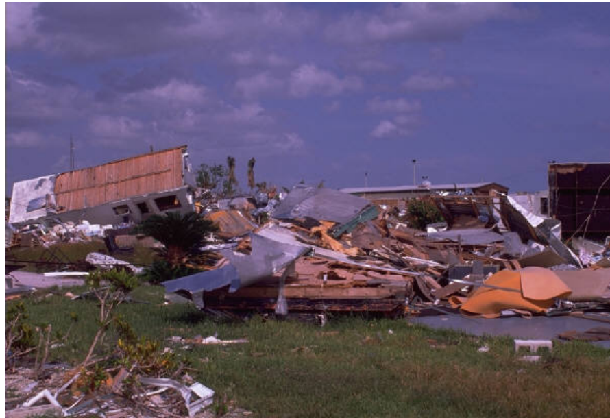
Hurricane damage typical of Florida and the Alabama Gulf Coast
